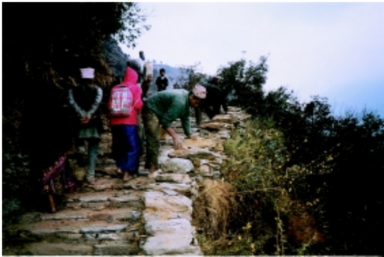
Community members of Tangram VDC, Baglung rehabilitating a foot trail
