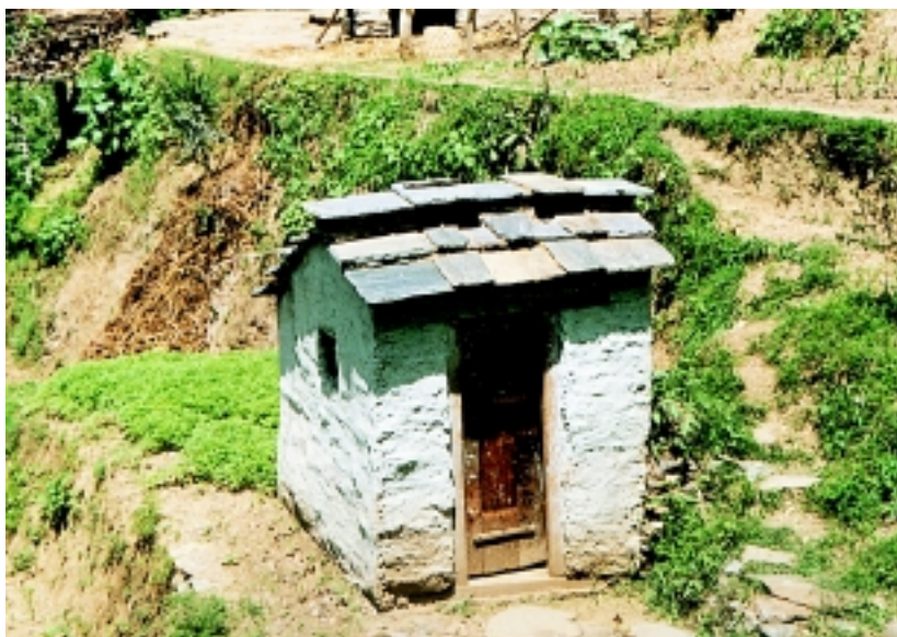
Toilet constructed in Ramaroshan VDC, Achham
